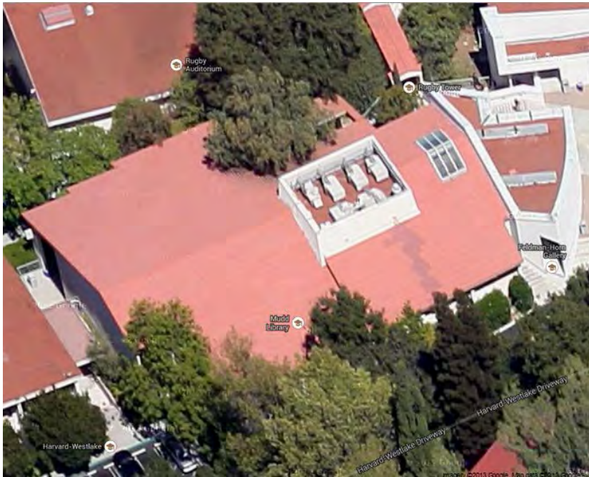
Mudd Library and Kutler Center site – Before Recent Renovation
